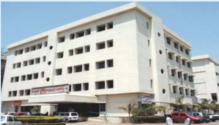
Bharati Hospital, Pune
